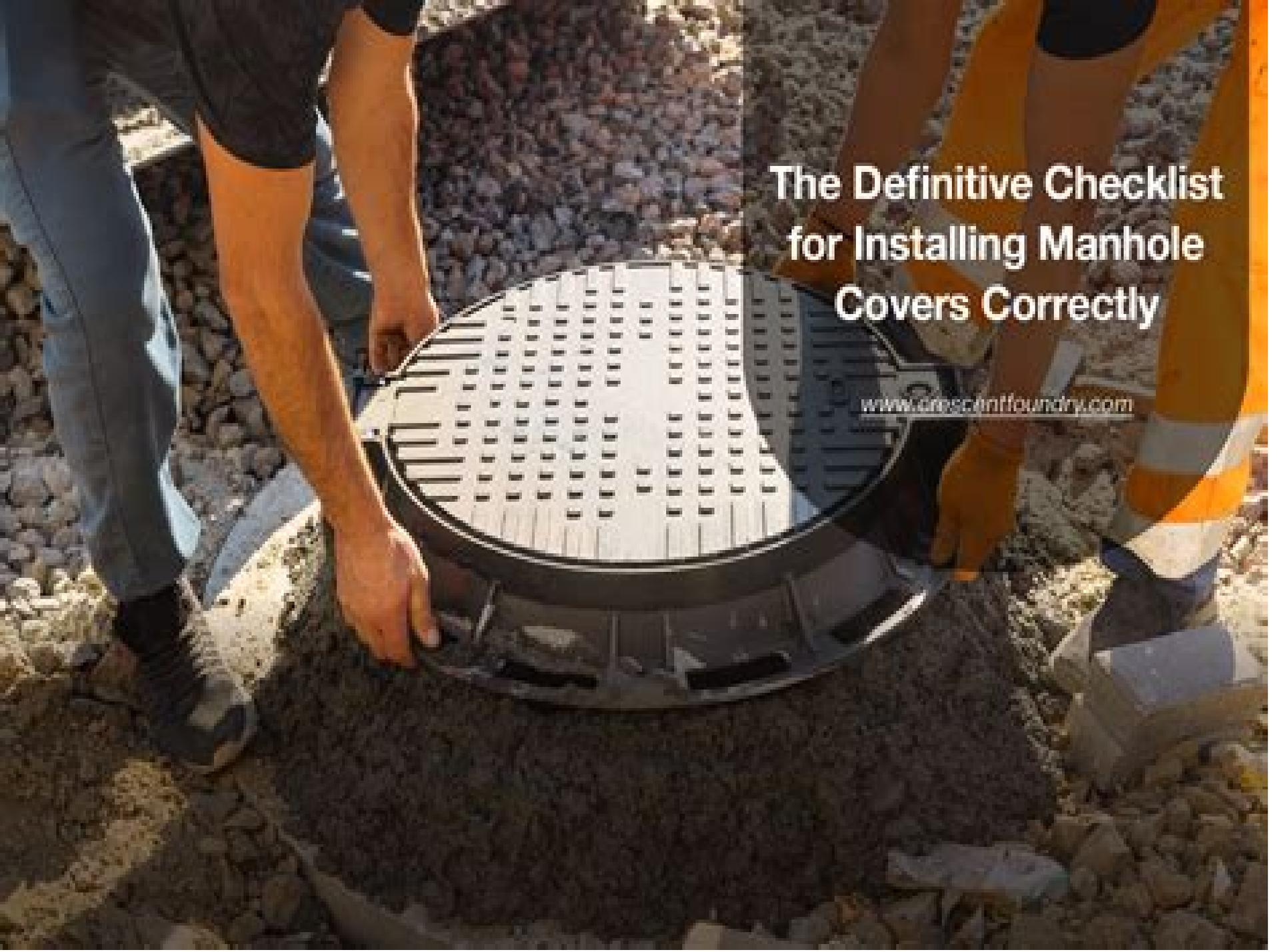
A high-angle photograph showing two workers in safety gear installing a large, circular, perforated metal manhole cover into a hole in the ground. The cover is being held by both workers, and the surrounding area is filled with gravel. The scene is brightly lit, suggesting an outdoor construction site.
